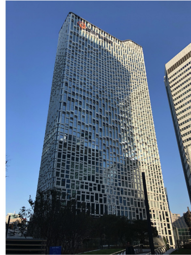
Fig. 26. Renovation of the Hanwha Headquarters building in Seoul, South Korea. The facade has been designed by UNStudio. This building shows an example of a facade in which the BIPV modules were not arranged vertically. The inclination of the modules increases the electrical yield. The concept and the ideas behind the design are explained in [115,116]. Pictures UNStudio, Amsterdam, the Netherlands.
