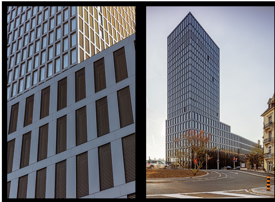
Fig. 22. Großpeter Tower, Basel, Switzerland. Around 10,000 thin-film solar modules in 450 different sizes were installed in this building. All facade orientations are covered with BIPV. The facade-integrated solar system has a total output of 440 kWp. Architecture: Burckhardt + Partner AG, Basel, Switzerland. BIPV Modules manufactured by Nice Solar Energy GmbH, Germany. Pictures ©NICE Solar Energy.
