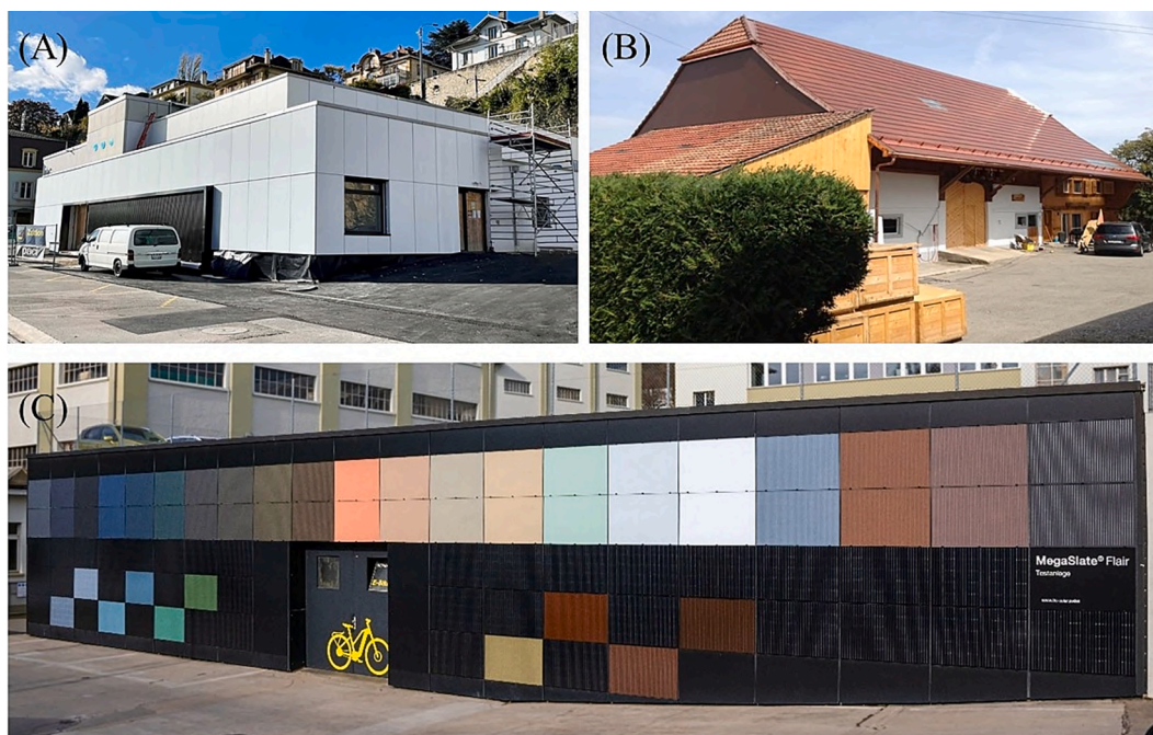
Fig. 1. (A) BIPV building made with a Solalexess nanotechnology white film. (B) With terracotta digital ceramic printing technology. Credit to Patrick Heistein. (C) Colored BIPV modules in a demonstrator in Bern. Courtesy of 3S Swiss Solar Solutions AG.
